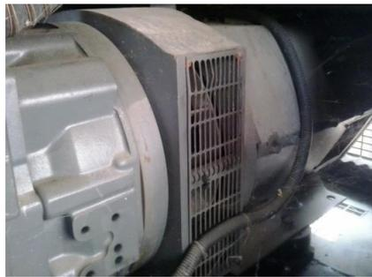
Gambar 3. Generator Sinkron 3 fasa merk Rexford
