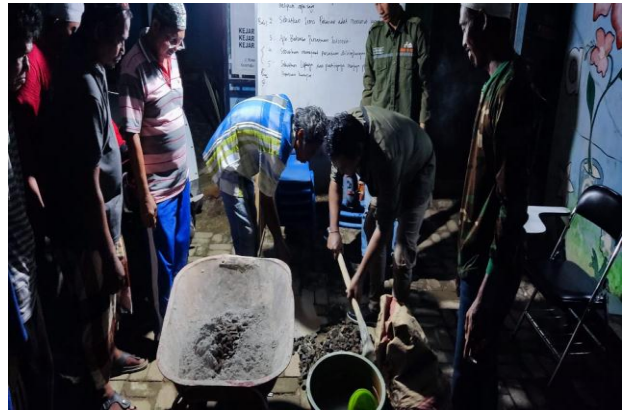
Gambar 3. Praktek Beton Normal
