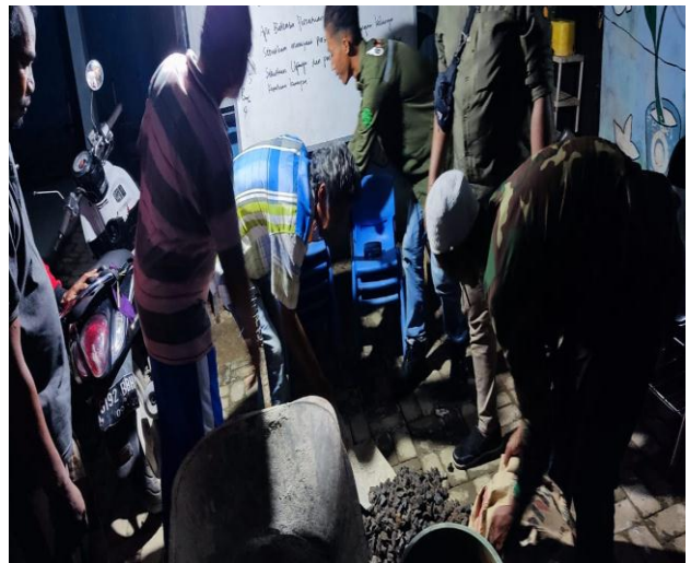
Gambar 5. Praktek Beton Porous Fly Ash
